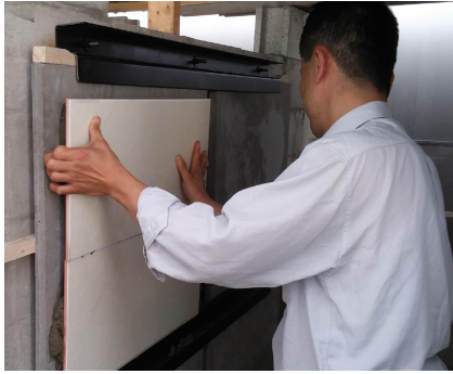
Figure 5. Sensual evaluation of tile direct setting constructivity
