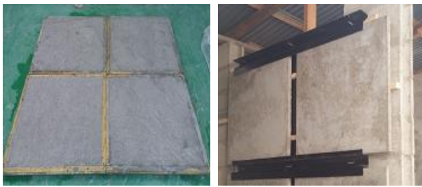
(a) preparing substrate concrete (b) setting substrate concrete
