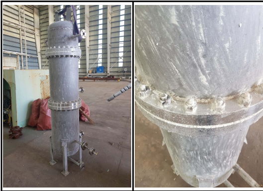
Fig. 7. Removed insulation of re-liquefaction drum.
