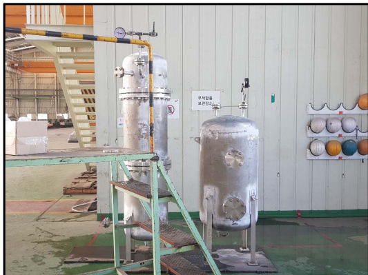
Fig. 2. Hydrostatic test of re-liquefaction drum.
