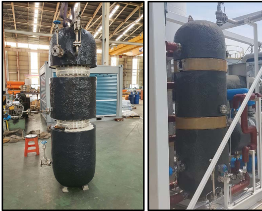
Fig. 10. Re-liquefaction drum after insulation construction change
