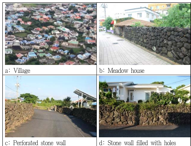
Figure 8. Houses, stone walls, alleys or narrow lanes (in villages) in Jeju Island
