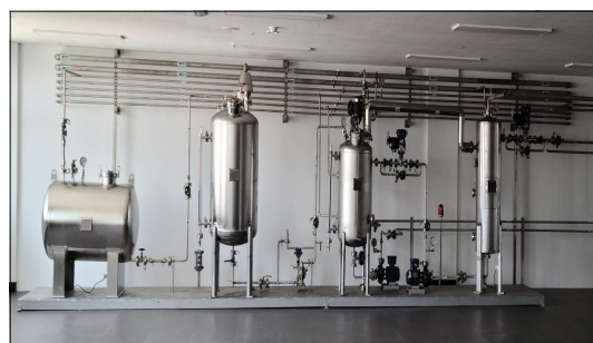
Fig. 2. Pilot Plant Site Photos
