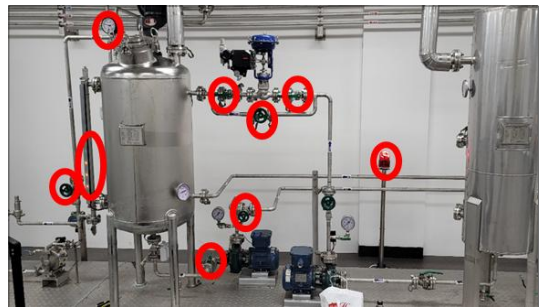
Fig. 10. Installation of remote control system
