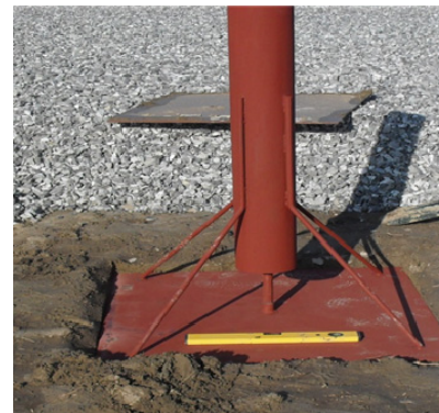
Fig. 3. Ground subsidence plate installation
