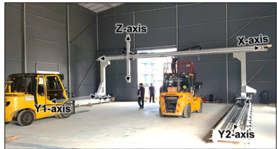
Fig. 1. Gantry System for Construction Scale Material Extrusion Additive Manufacturing
