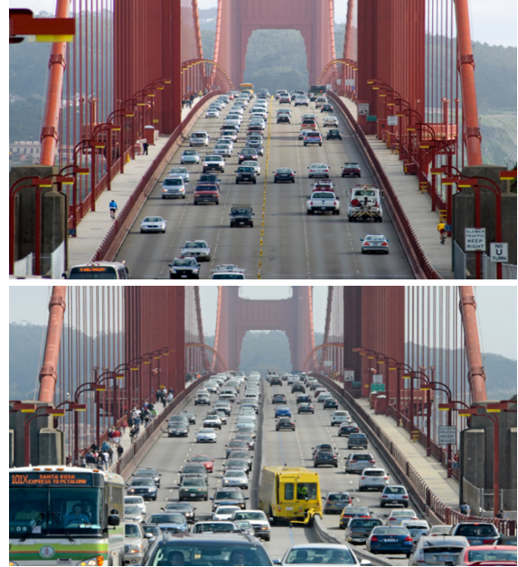
Fig. 1. Traffic Control on Golden Gate Bridge Before (left) and After BTS (right) (Kang and Chung, 2020)
