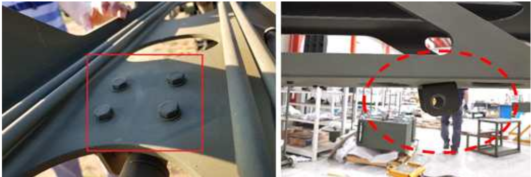
Figure 4. Rear Rail Deformation
