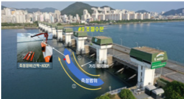
Figure 1. Measuring discharge through gate using ADCP.
