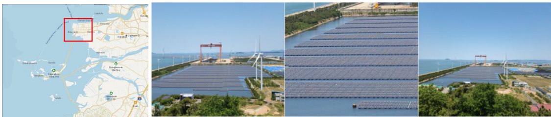
Fig. 2. Floating Solar Power Location Map and Photo
