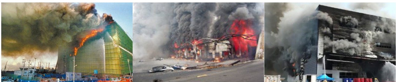
(a) Busan Refrigeration Warehouse New Construction Fire ('98.10.29)
