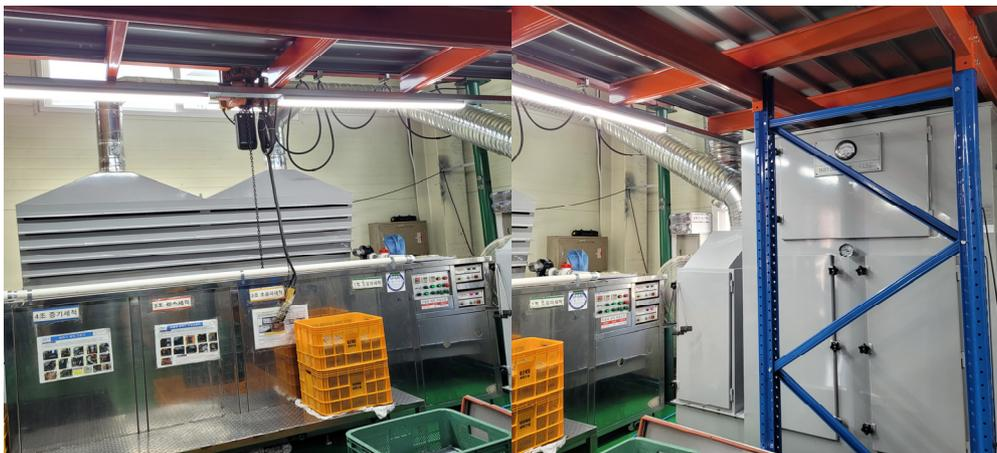
Figure 1. Local exhaust system and drying rack
